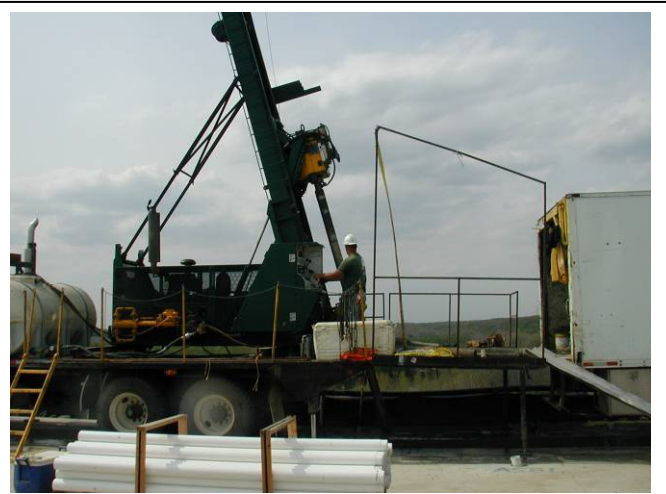
Figure 5: Sonic Drilling Rig
